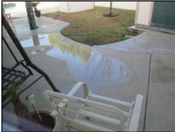
Ponding water-poor drainage
