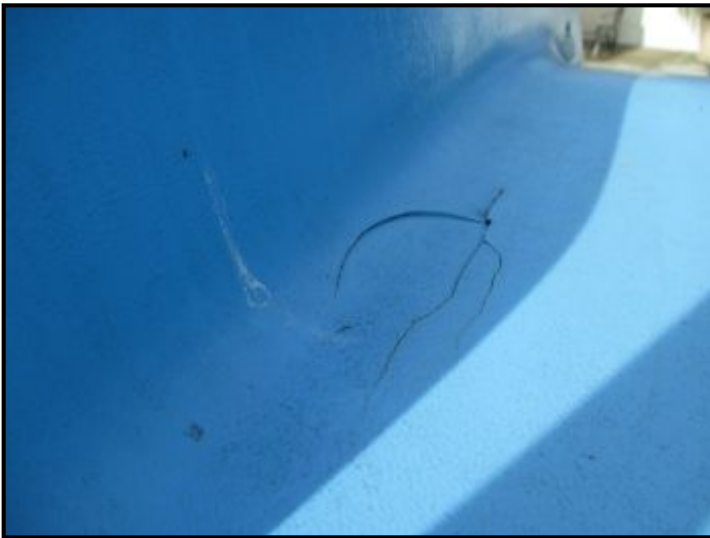
Damaged Pool Slide
